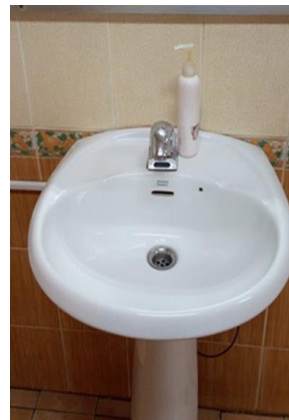
Washbasins water-saving sensor taps
